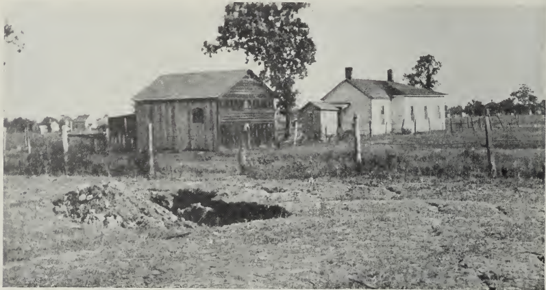
FIG. 36.—Pit hole and cracks caused by mining at a shallow depth near Streator. Mine rock near the hole has been hauled for filling; the surface will then be dressed with soil.
